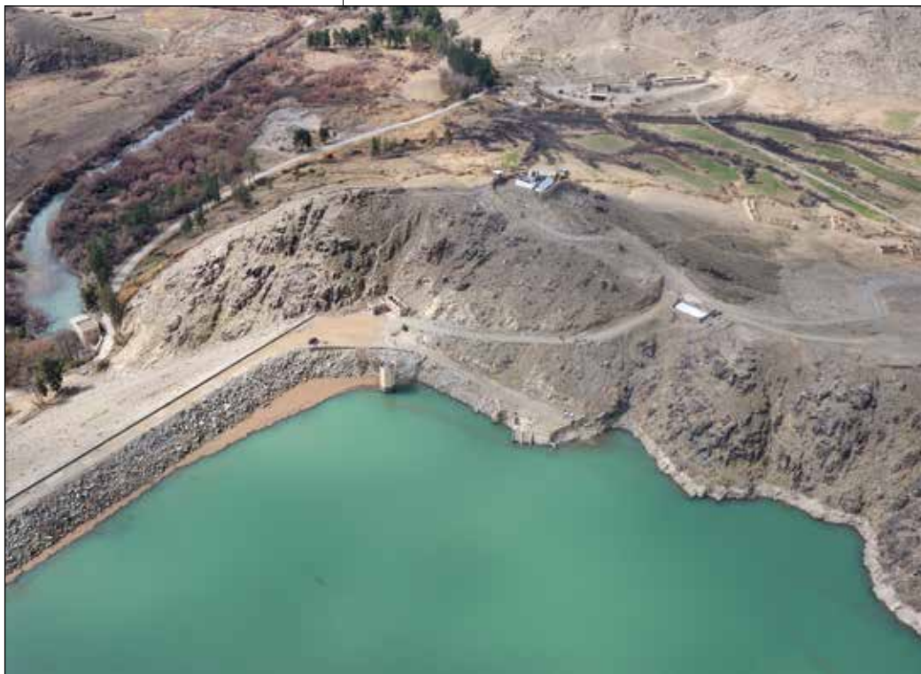
The Dahla Dam and irrigation system, one of three Canadian signature projects in Afghanistan.
